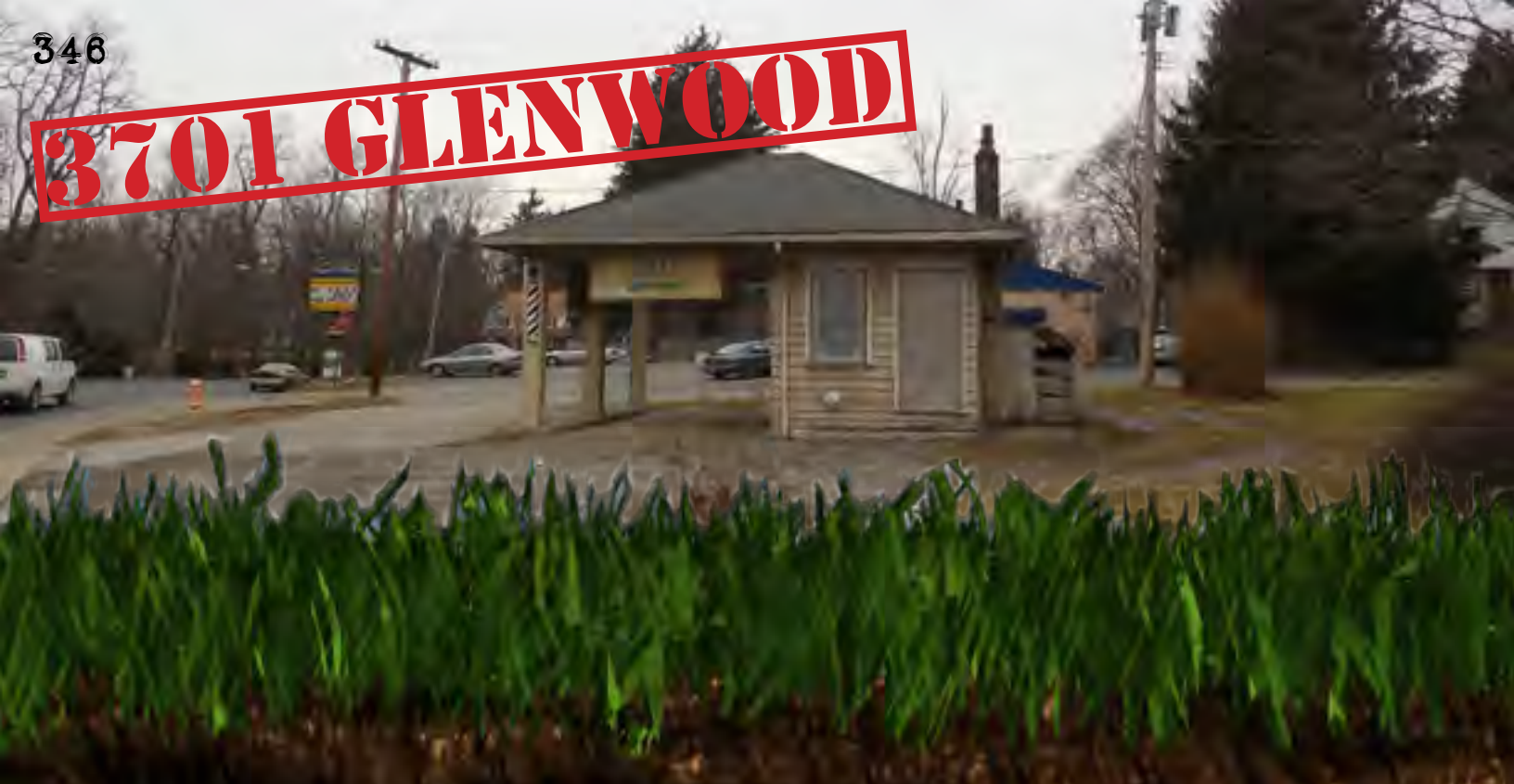
Former Gas Station
